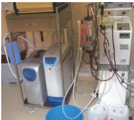
Figure 6 – the individual water treatment system
