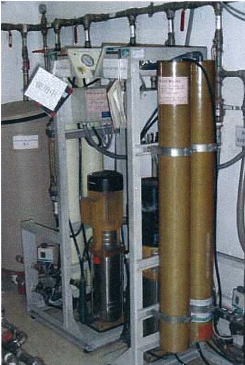
Figure 3: An advanced water treatment system to provide high quality, pyrogens free water for HD.
